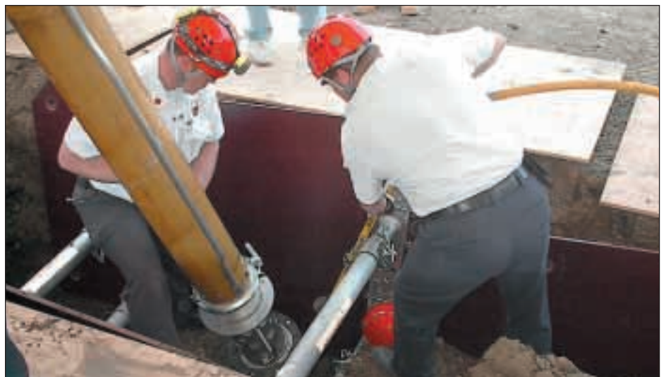
Air tools pulverize the soil for vacuum excavation.
